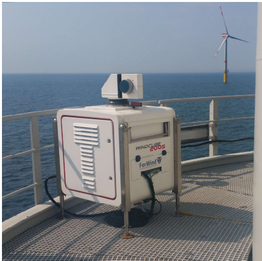
Figure 3. Lidar system Windcube 200S on the transition piece of wind turbine GT58 in the offshore wind farm Global Tech I. On the right side of the image the tower of the turbine is visible while turbine GT51 northwest of GT58 can be seen in the background (cf. GT I layout in Fig. 2) (Stephan Voß, ForWind).
